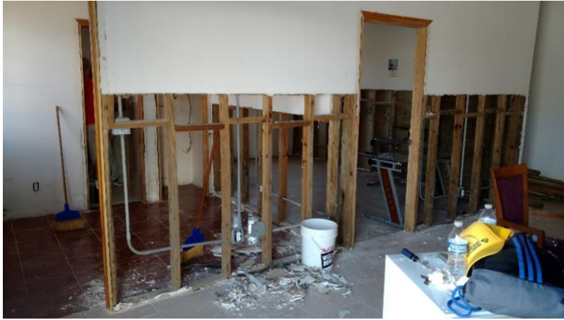
Team 1 removed moldy sheetrock & did a lot of cleaning up
